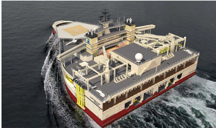
Figure 2: The configuration of a modern seismic ship [4]
