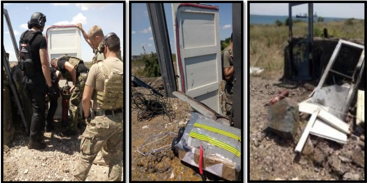
Figure 2. a) & b) Creation of breach in a wooden door with an explosive load made of a detonating wick and an double adhesive tape and c) the effect obtained
