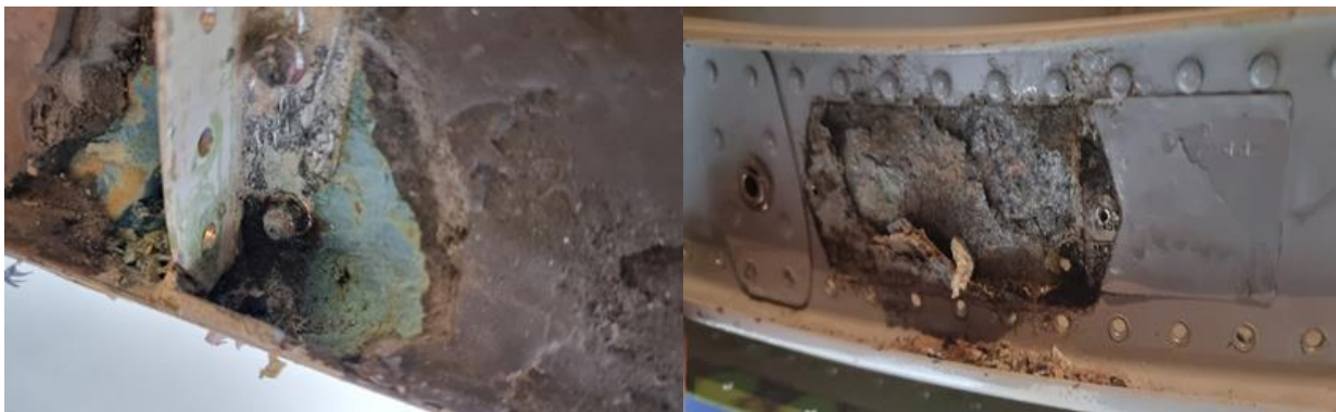
Figure 2. Corroded aircraft structural components
