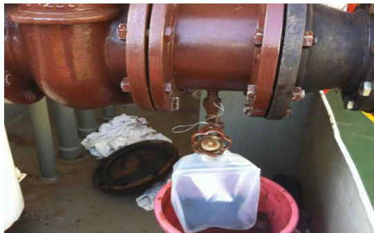
Figure 1 – Drip type fuel bunker sampler [1]
