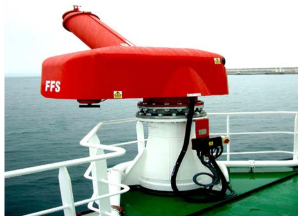
Figure 12 - Fire-fighting remotely controlled monitors
