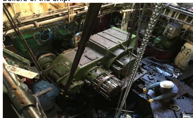
Figure 5 -Removing and extraction of the ME gearbox
