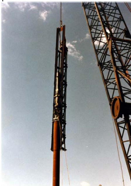
Figure 1 A standard pile driving operations ( www.vulcanhammer.info )
